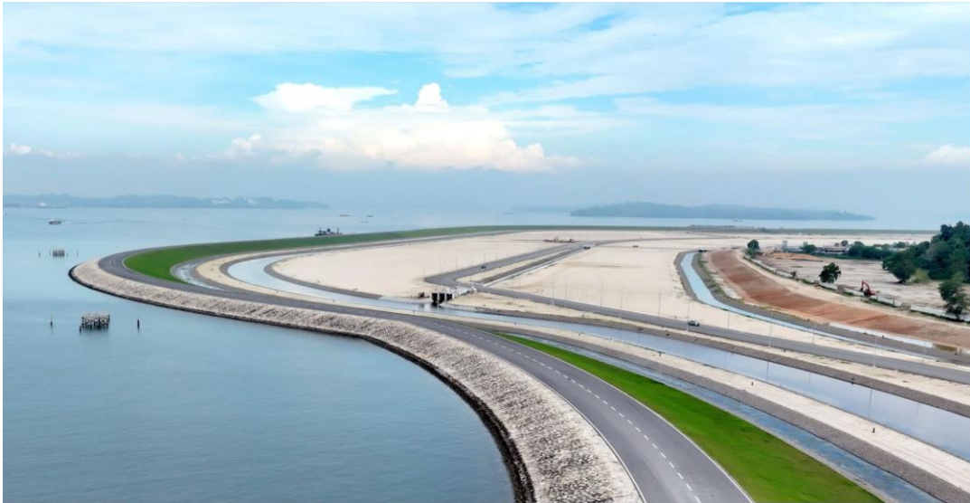
Natural materials are used on both sides of the coastal dike. (Credit: HDB)
