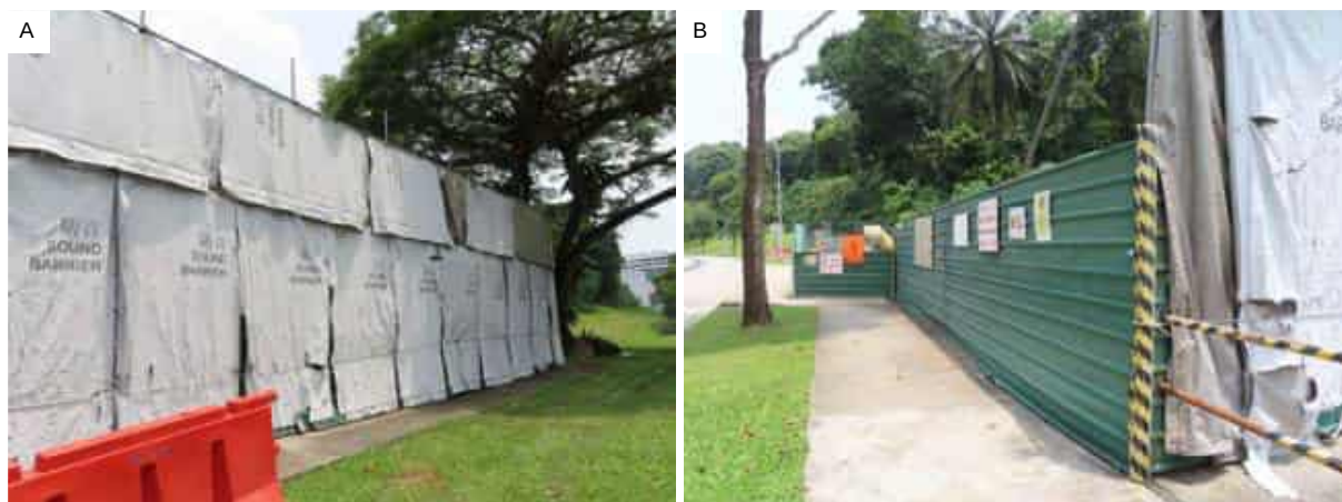
Figure 6.4.10 (A–B) Others (Construction) in the Study Area
