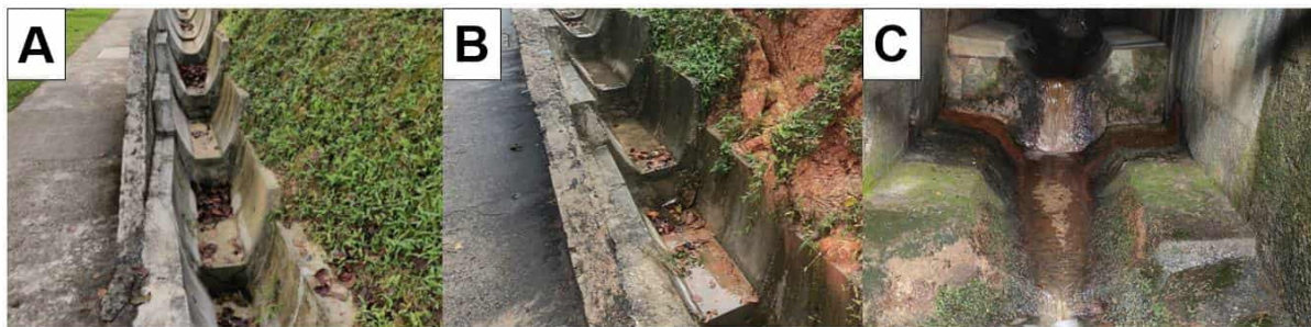
Figure 6.5.2 Photographs of drain D1 during (A) dry weather; (B) wet weather conditions; and (C) discharge point during wet weather conditions (underground)
