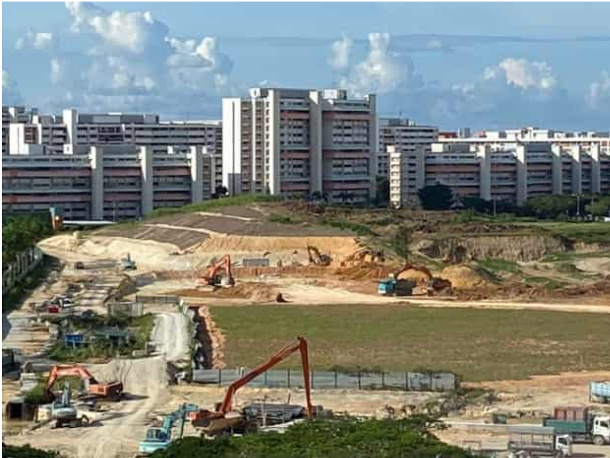
Figure 3.3.2 An example of site levelling at construction worksite in Singapore (AECOM®)
