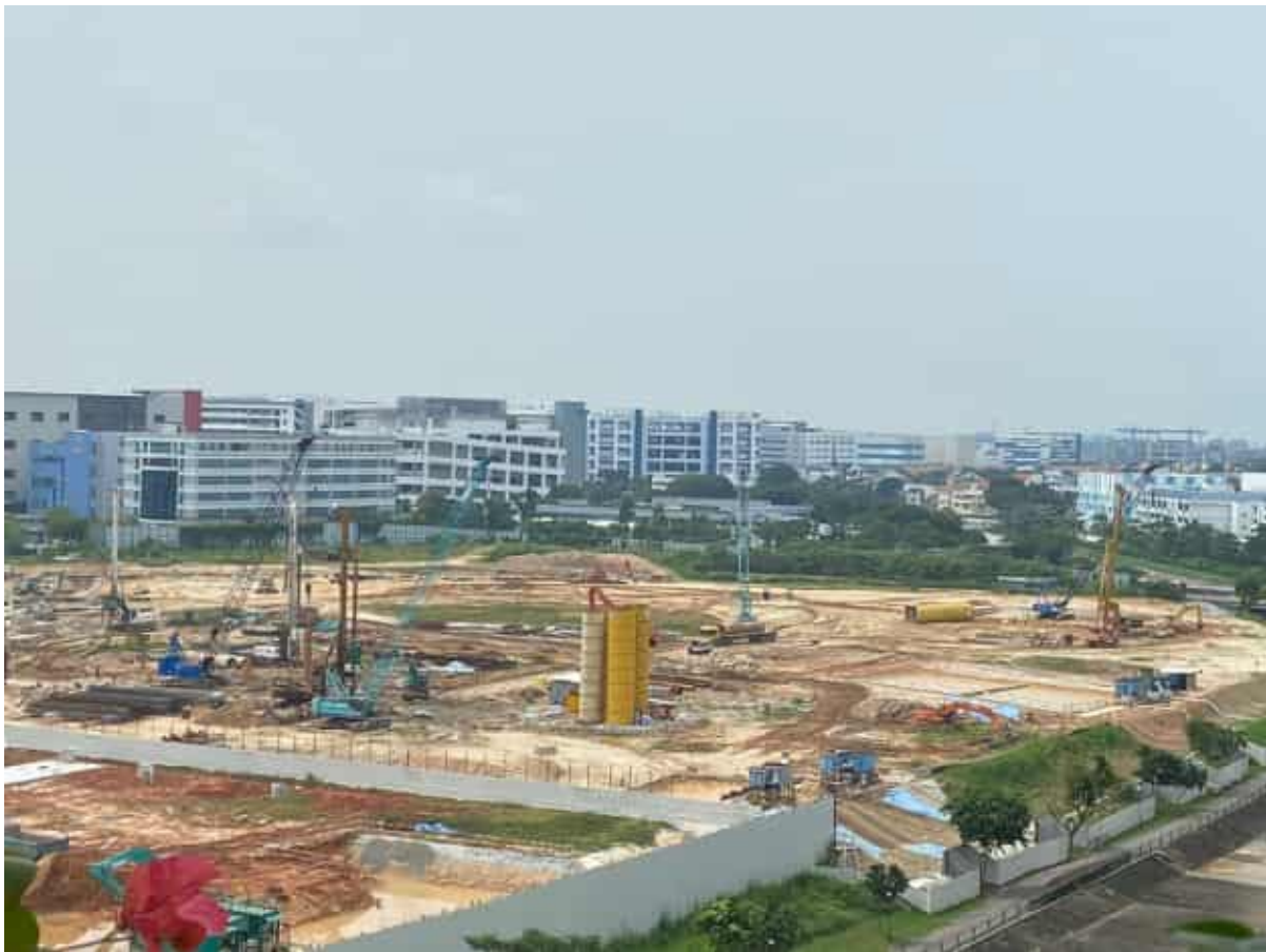
Figure 3.3.3 An example of piling/ foundation works in Singapore (AECOM ©)
