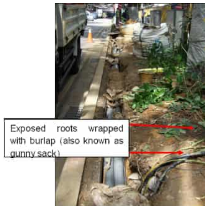
Figure 9: Tunneling under roots.
