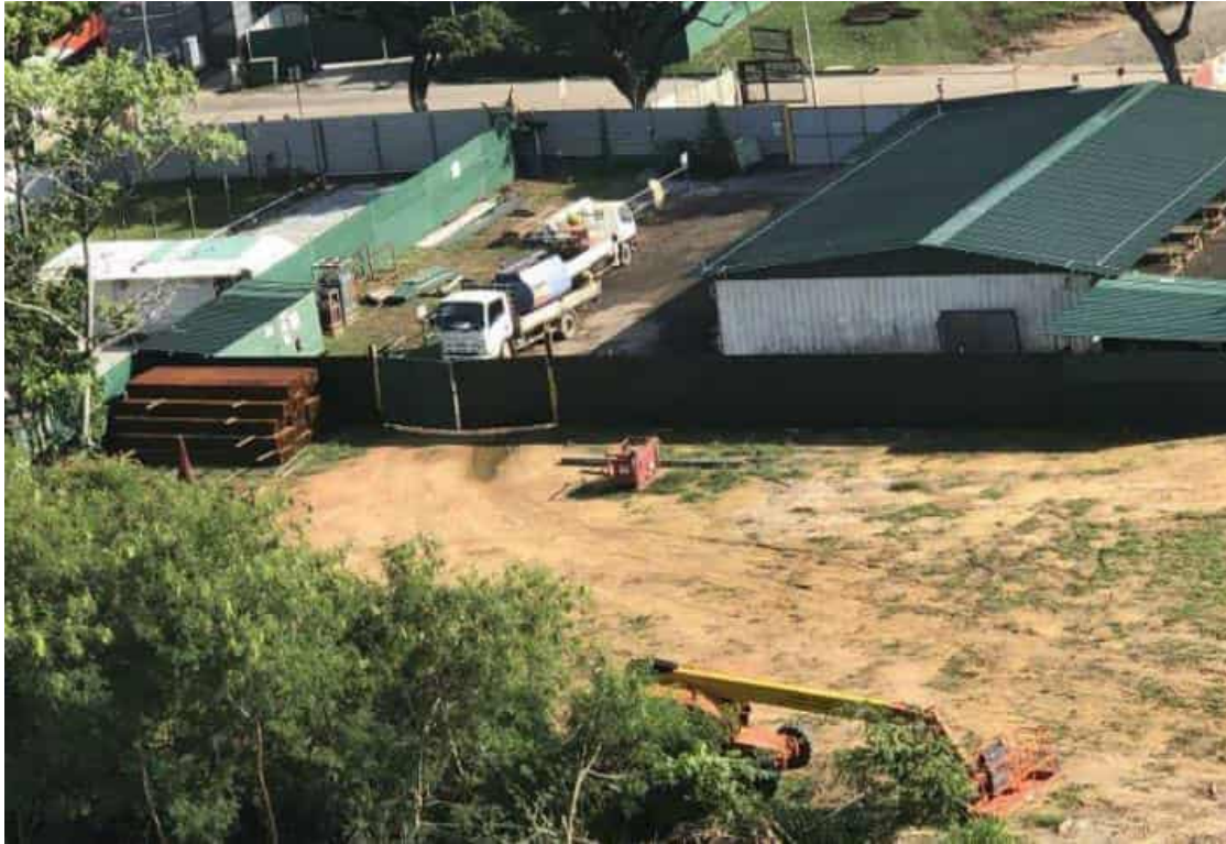
Figure 3.3.1 An example of site clearance at construction worksite in Singapore (Construction Site near Bedok Reservoir, Digital Photograph)
