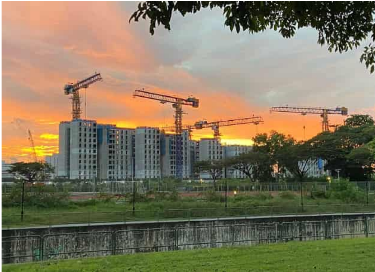
Figure 3.3.4 An example of superstructure construction works in Singapore (AECOM ©)
