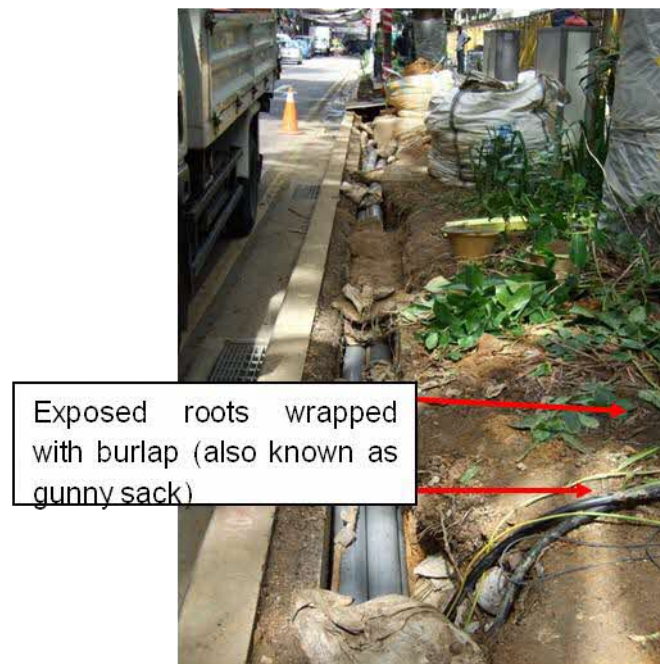
Figure 9: Tunneling under roots.
