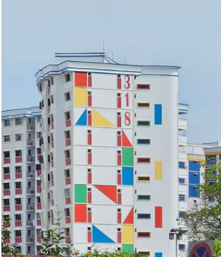
Blocks with roofs featuring the distinctive blue and white stripes of sailors, and colourful triangles on the façade referencing maritime signal flags
