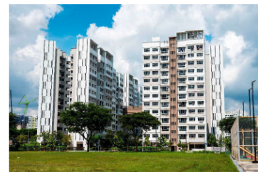
Facades with distinct brown vertical pattern at EastGlen @ Canberra
