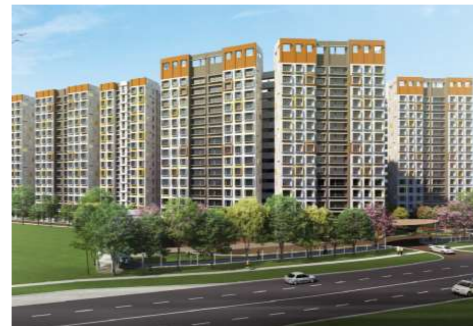
Light and porous elements in the facade design in artist's impression of Garden Bloom @ Tengah
