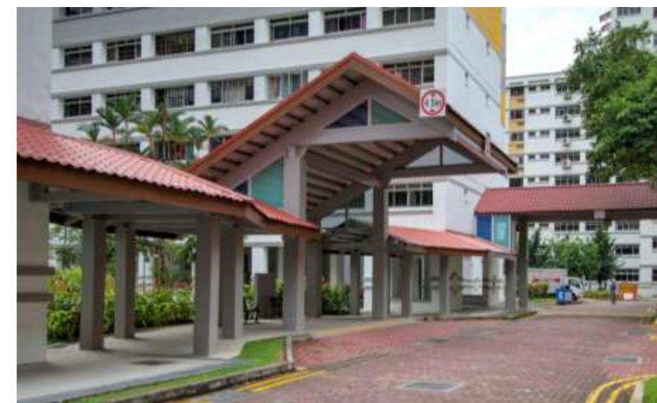
Careful interfacing between linkways and a new drop-off porch added to an existing HDB precinct (example from Choa Chu Kang North 7)
