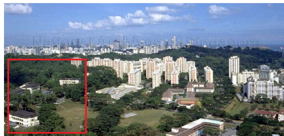
Fig. 2.2.64 1990 View of the now demolished office and accommodation blocks (in red) with Telok Blangah in the background. Source: Ministry of Information and the Arts Collection, courtesy of National Archives of Singapore
