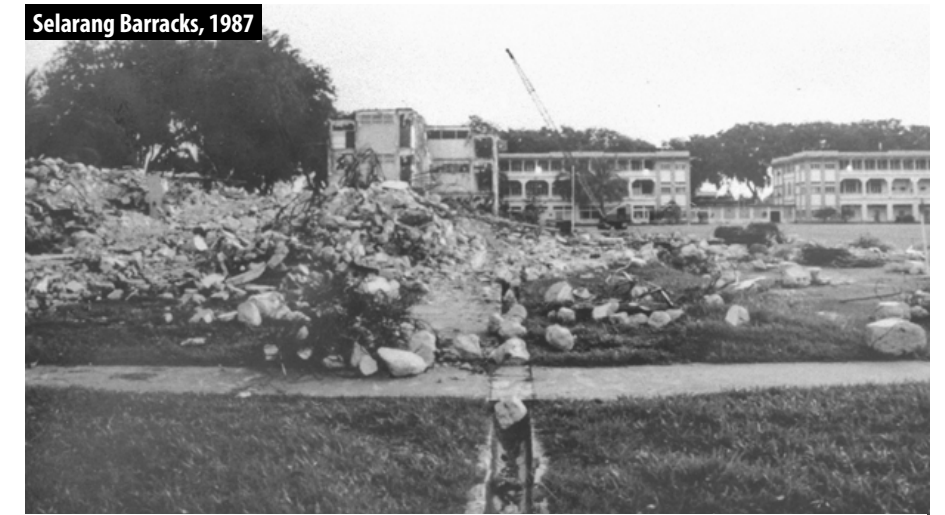
Fig. 3.27 Demolition of Selangor Barracks in 1987. Source: Ministry of Defence Collection courtesy of National Archives of Singapore
