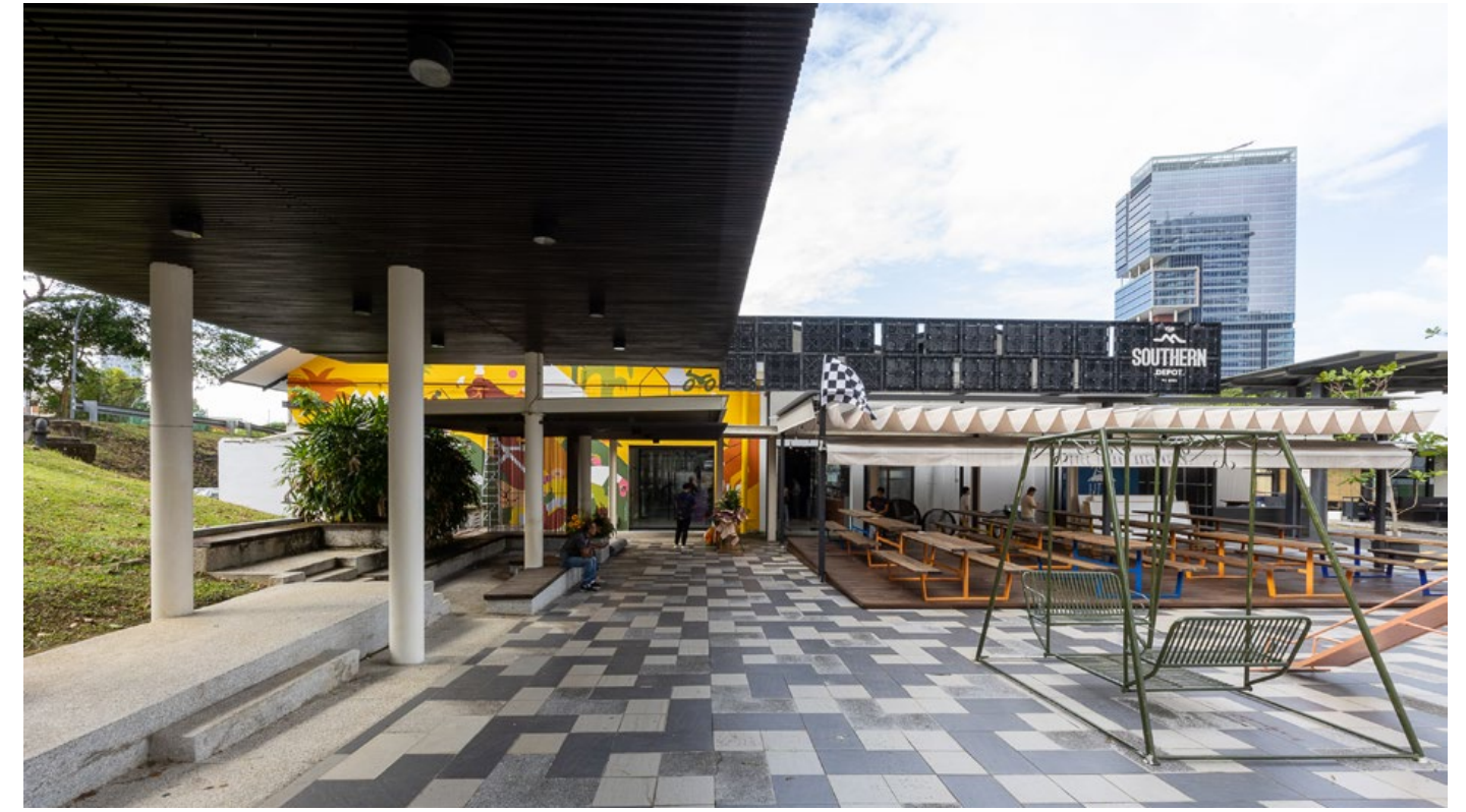
Fig. 2.2.95 43 Malan Road at Gillman Barracks which houses The Southern Depot today. Source: Studio Lapis Collection
