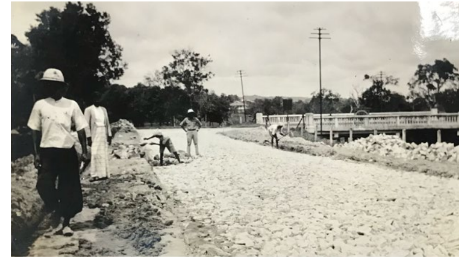
Fig. 2.2.10 1935 Junction of Depot Road with Alexandra Road ready for carpet. Source: The Royal Engineers Museum; Collection No. 6/20.
