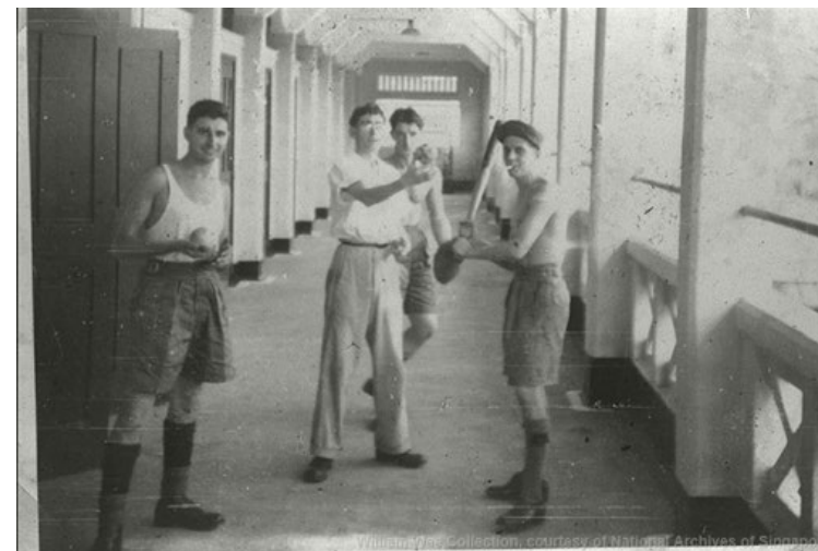
Fig. 2.2.35 Corridors of Gillman Barracks. Source: William Wee Collection, courtesy of National Archives of Singapore
