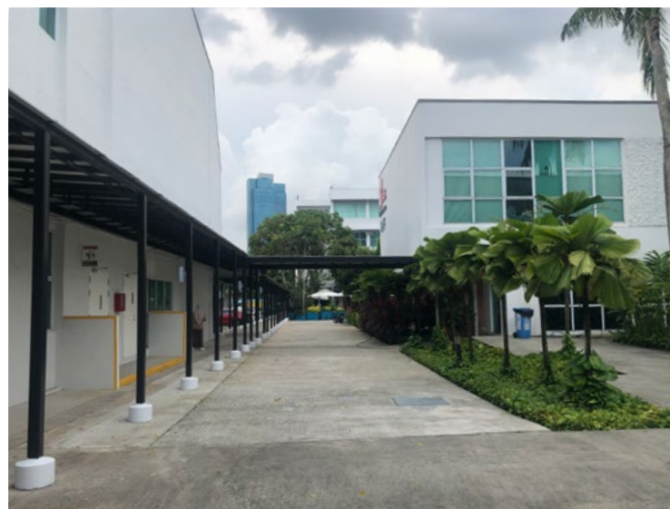
Fig. 5.9.7 Present-day hardscape and sheltered walkway connecting the blocks. Source: Studio Lapis Collection.
