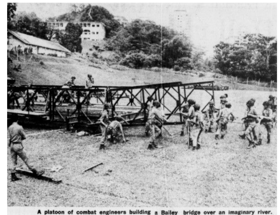
Fig. 2.2.61 SAF Combat Engineers building a Bailey bridge during training in 1978. Source: The Straits Times © SPH Media Limited. Reprinted with permission.
