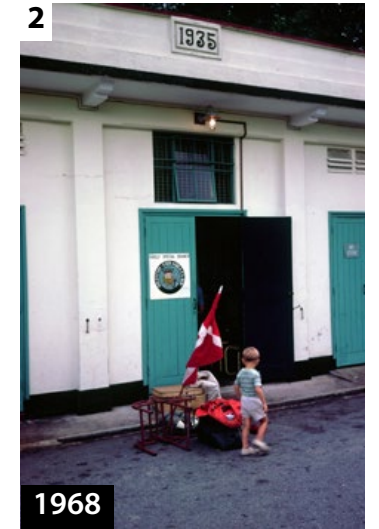
Fig. 5.4.7 1968 Facade of 38 Malan Road. Source: John C Young Collection, courtesy of National Archives of Singapore
