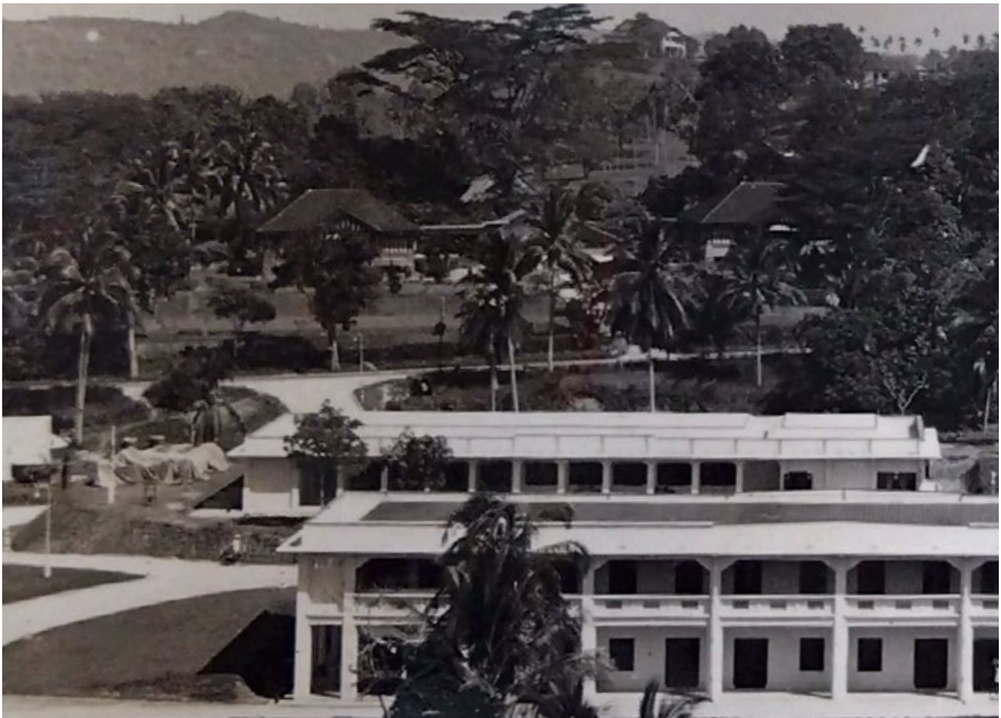
Fig. 5.5.14 View of 5 Lock Road, the building nearest to the entrance of Gillman Barracks when approached from Alexandra Road. Visible in the foreground and situated across the building is 6 Lock Road. Source: Courtesy of National Army Museum, London
