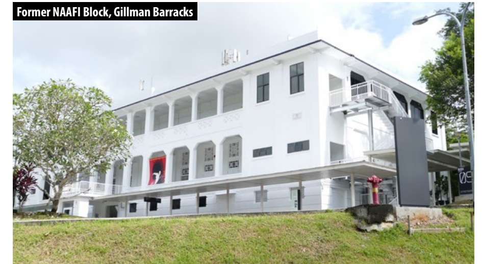
Fig. 3.30 Former NAAFI Block at Gillman Barracks. It is an extremely rare representation of interwar military barracks in Singapore. Source: Studio Lapis
