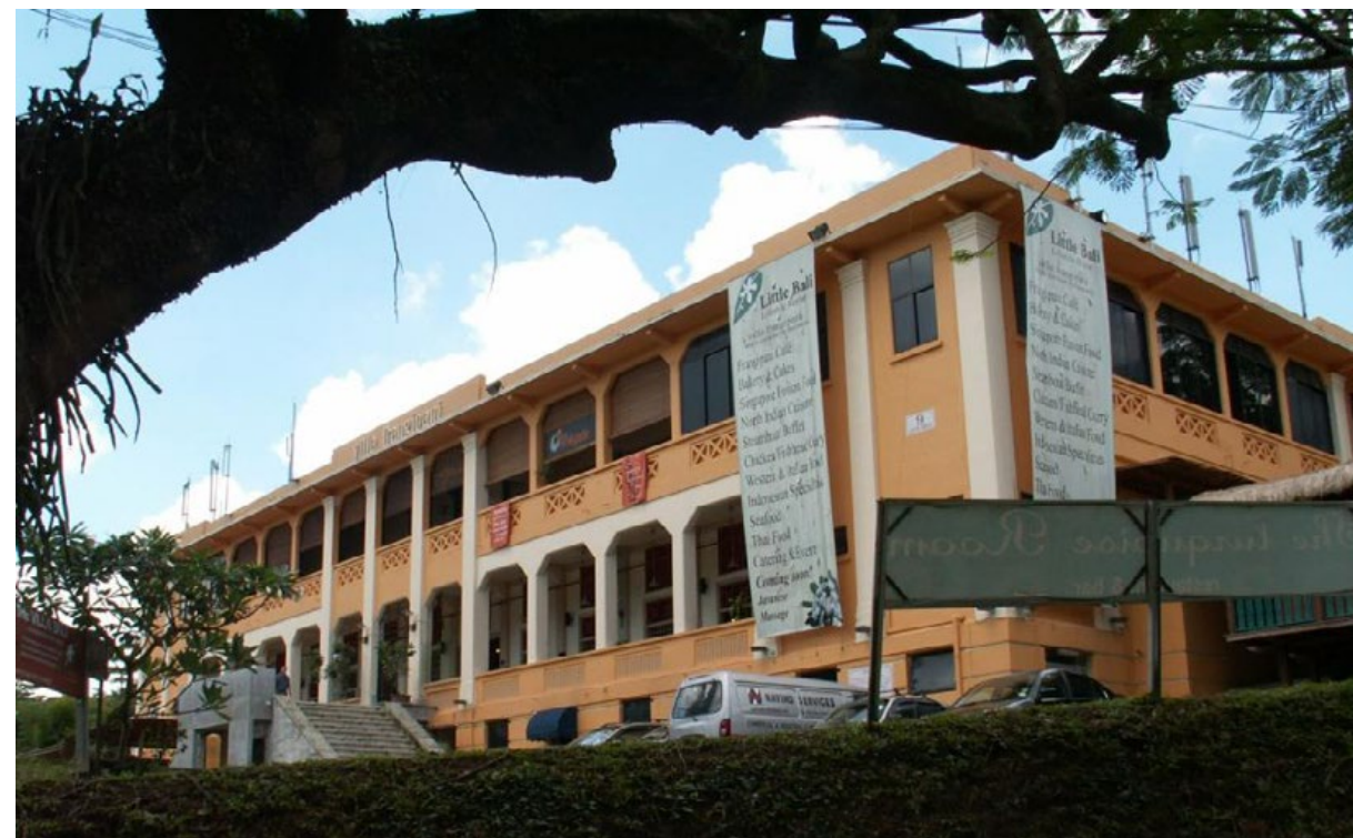
[Top] Fig. 2.2.82 9 Lock Road seen from Lock Road along its eastern rear facade, when it housed master tenant Villa Frangipani. Source: Xin Li [Bottom] Fig. 2.2.83 Little Bali set up at 9 Lock Road, which hosted F&B spaces. Source: Lam Chun See
