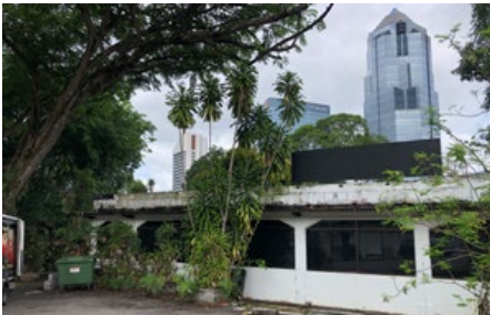
[8] Former Orderly Room - 8 Lock Road
