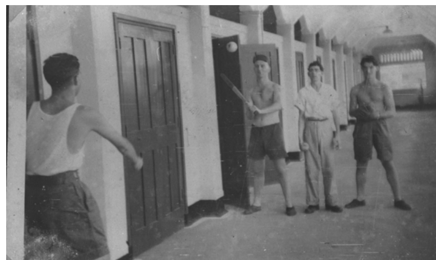
Fig. 7.21 Corridors of Gillman Barracks. Source: William Wee Collection, courtesy of National Archives of Singapore
