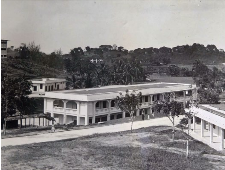
Fig. 5.5.15 Former quartermaster's store at 6 Lock Road seen along the main arterial spine of Lock Road. Source: Courtesy of National Army Museum, London
