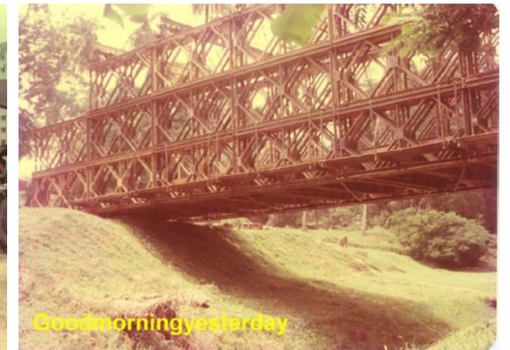
Fig. 5.1.11 1977, Bailey Bridge, Gillman Barracks. Source: Lam Chun See.
