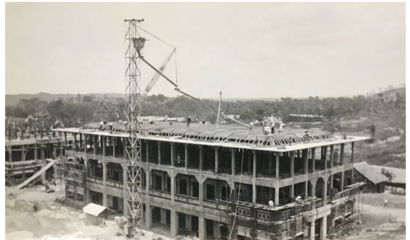
Fig. 5.1.9 1935, placing reinforcement and tower for pouring concrete at high level roof of Block D. Source: The Royal Engineers Museum; Collection No. 6/20.
