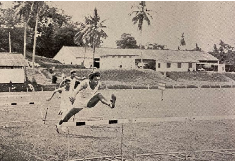
Fig. 5.4.12 1963 view of 47 Malan Road set in the background. The building overlooks the recreational field where Alexandra Grammar School students participate in the Pasir Panjang District Meet. Source: Alexandra Grammar School
