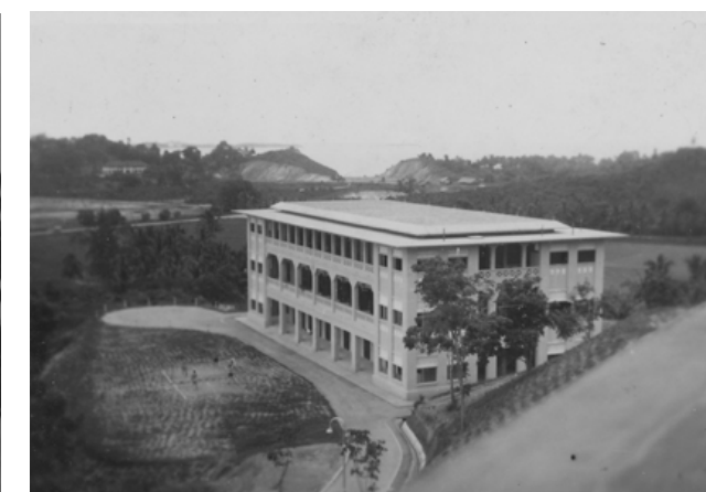
[Left] Fig. 2.2.17 View looking down Malan Road towards the hill where the company offices and blocks were sited
