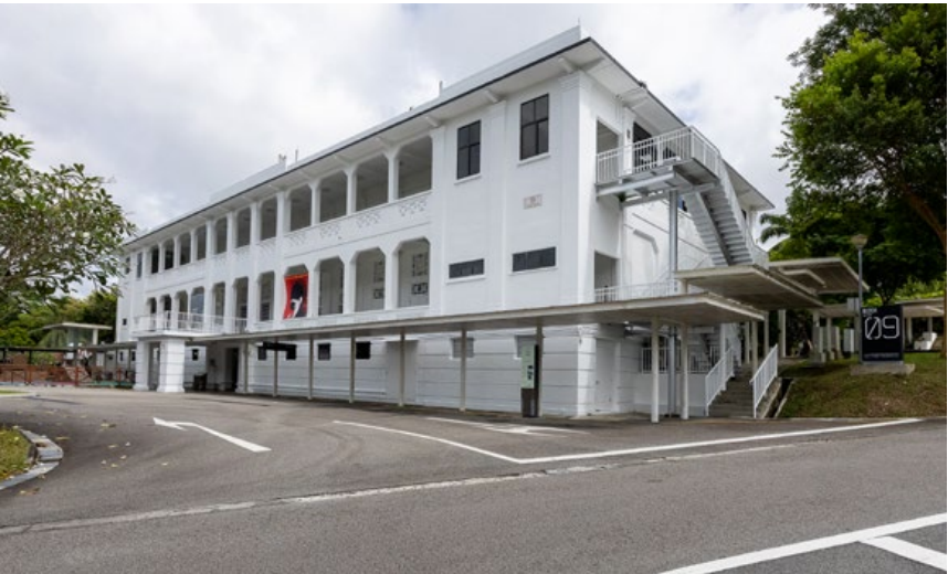
Fig. 5.5.18 View of 9 Lock Road perched at one of the highest points along Lock Road. Source: Studio Lapis Collection
