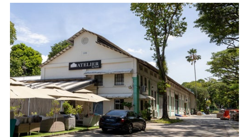
Fig. 2.3.6 View of 1936-built storage facility at the former Royal Army Ordnance Corps depot built contemporaneously with Gillman Barracks. Source: Studio Lapis Collection
