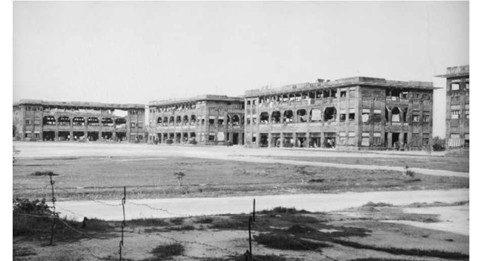
Fig. 3.24 The buildings at Roberts Barracks feature a flat RC roof construction, c. 1942. All but Block 151, which houses the Changi Murals by Stanley Warren, of Roberts Barracks have been demolished. Source: John Rosson via Australian War Memorial
