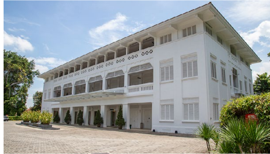
Fig. 3.23 The buildings of the former Kitchener Barracks, now along Hendon Road, have undergone adaptive reuse thus retaining a representation of interwar military barracks with pitched roofs in Singapore. Source: Jerome Lim
