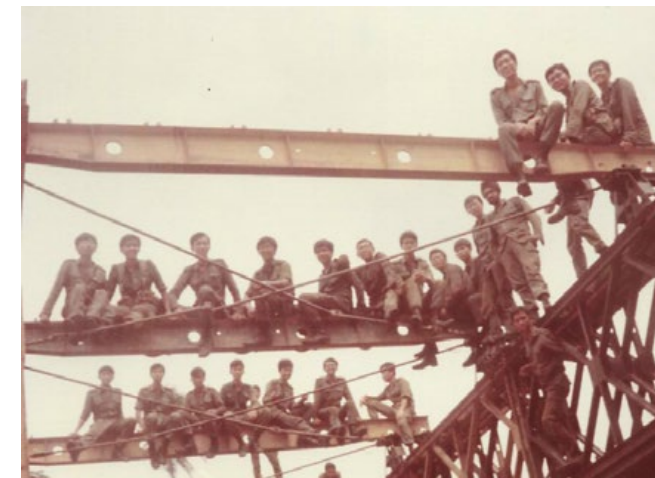
Fig. 5.1.14 1977 Bailey Bridge and combat engineers, Gillman Barracks. Source: Lam Chun See.
