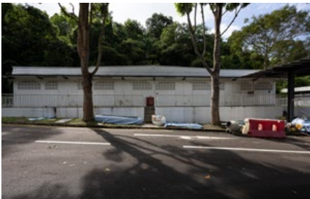
[14] Medical Inspection Room - 37 Malan Road
