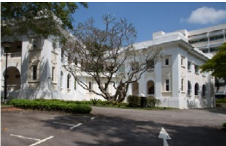
[11] Former Officers' Mess - 10 Hyderabad Road. Source: Jerome Lim
