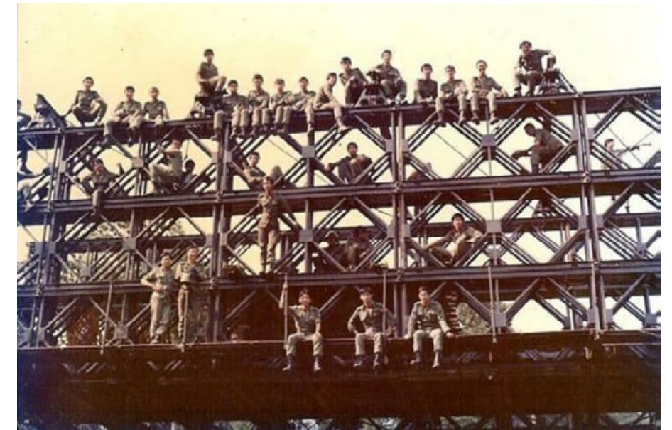
Fig. 4.27 Construction of the Acro Panel bridge. Source: John Lynn
