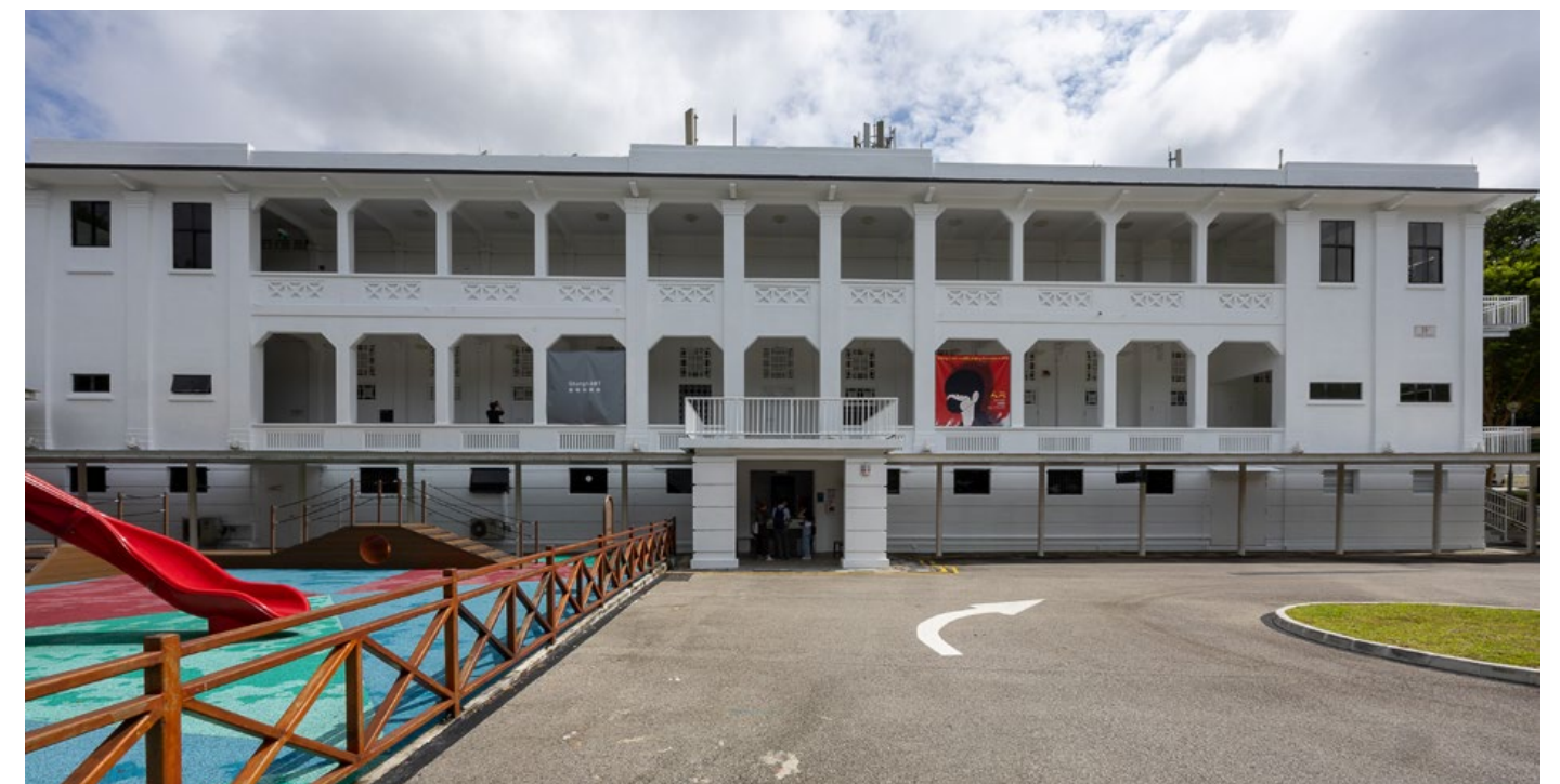
Fig. 2.2.96 9 Lock Road at Gillman Barracks today. Source: Studio Lapis Collection
