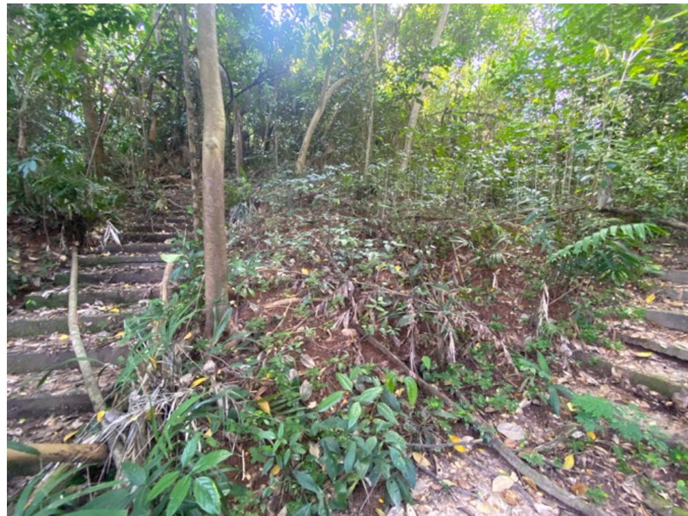
Fig. 5.4.3 Present-day view of the staircase on the slope of Barrack Hill which has been partially demolished and the existing portions heavily overgrown and now a secondary forest. Source: Studio Lapis Collection.
