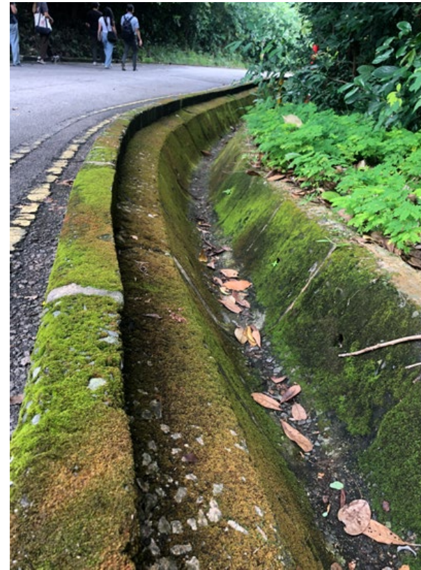
Fig. 5.6.3 Present-day view of the drains along Preston Road. Source: Studio Lapis Collection.
