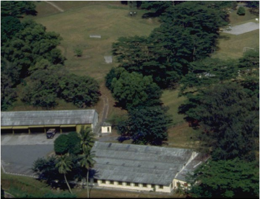
Fig. 5.4.11 1990 Aerial photo of 43 Malan Road in the foreground, with view of historic fenestration along its west-facing facade. Source: Ministry of Information and the Arts Collection via National Archives of Singapore
