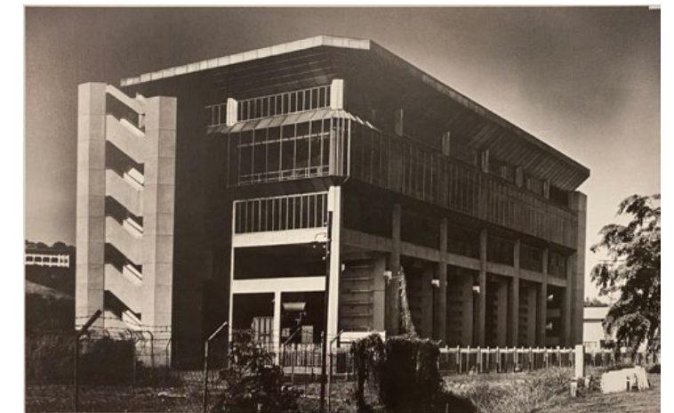
Fig. 5.10.3 1977 View of the 66kv substation commissioned by the Public Utilities Board and used to house electrical transformers and ancillary apparatus. Source: Kumpulan Akitek.
