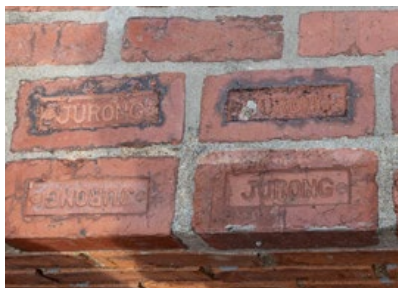
Fig. 5.8.19 Jurong Brickworks used across the central plaza. Source: Studio Lapis Collection
