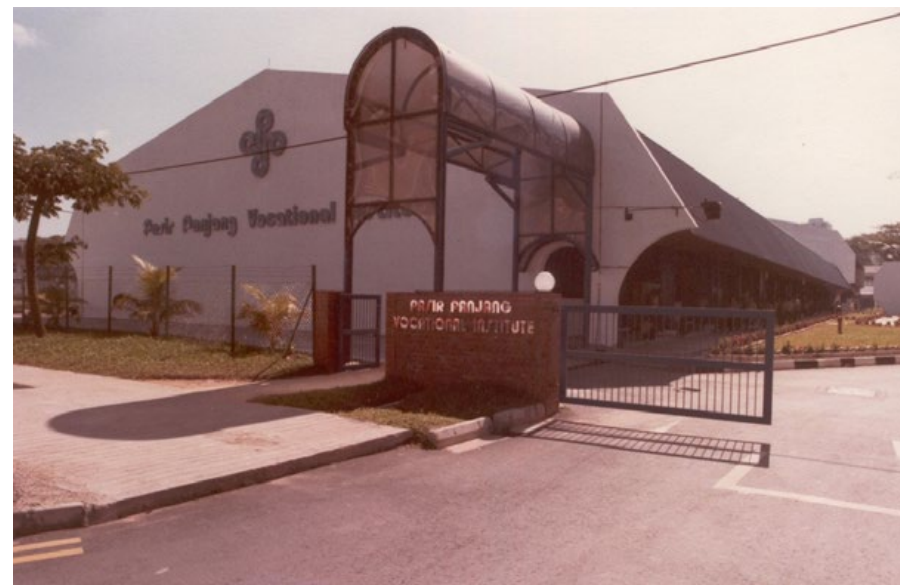
Fig. 2.2.74 Entrance of Pasir Panjang Vocational Institute. Source: Institute of Technical Education
