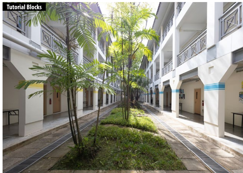
Fig. 5.8.21 Courtyard space between the tutorial blocks, where the rhythm and profiles of the columns and railings have been retained. Source: Studio Lapis Collection
