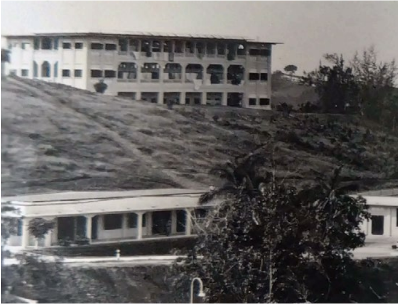
Fig. 5.4.14 c.1935-1938 View from Lock Road looking up towards Barrack Hill. The building on the left at the foot of Barrack Hill is 37 Malan Road. Source: Courtesy of National Army Museum, London
