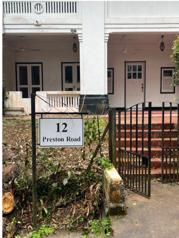
Fig. 5.6.1 Present-day view of address signage, same used across SLA owned properties. Source: Studio Lapis Collection.
