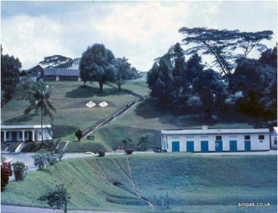
Fig. 5.4.13 1960s view of from Malan Road looking up towards Barrack Hill. 38 Malan Road is the building on the right with teal coloured doors during its use as the FARELF Sub Aqua Club building. Source: Paul Cook
