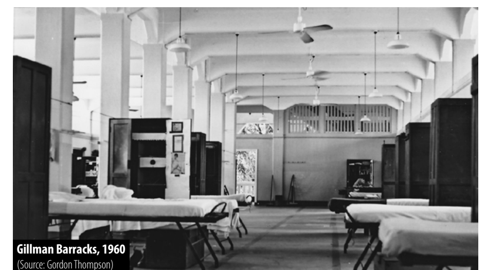
Fig. 3.19 The haunched beams in the RC frame structure can be seen on the facade and internal spaces of the interwar military barracks. With an additional structural bay provided to shorten the barrack block, a row of columns can be seen in the barrack room.
