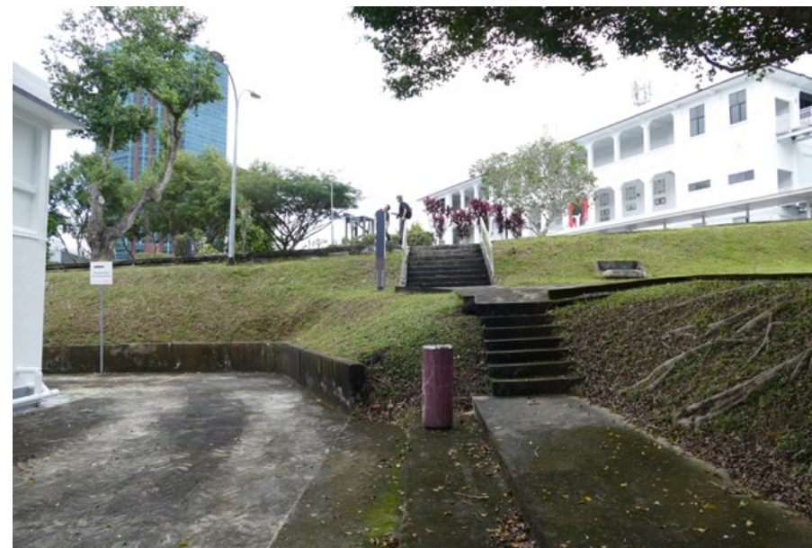
Fig. 5.5.7 The blocks of roads in this cluster are pedestrian friendly with pathways and steps (sheltered and unsheltered) that provide circulation between the various levels. Source: Studio Lapis Collection
