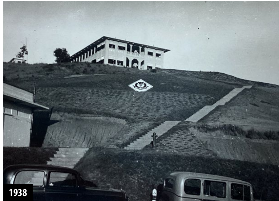
Fig. 5.4.1 1938, view of the slope of Barrack Hill from Malan Road. Visible in the frame is the military insignia, staircase and newly turfed slopes just after the completion of Gillman Barracks. Source: Courtesy of National Army Museum, London.
